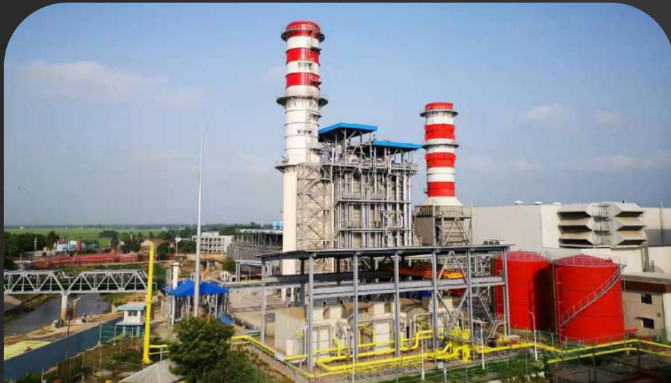
Ashuganj 400MW Combined Cycle Power Plant, Bangladesh
