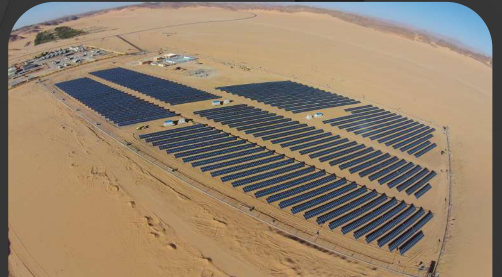
25 MW photovoltaic power plants, Algeria
