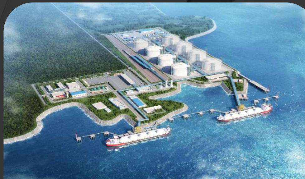
Whole-process Consulting Service for an LNG Project in Taizhou, Zhejiang
