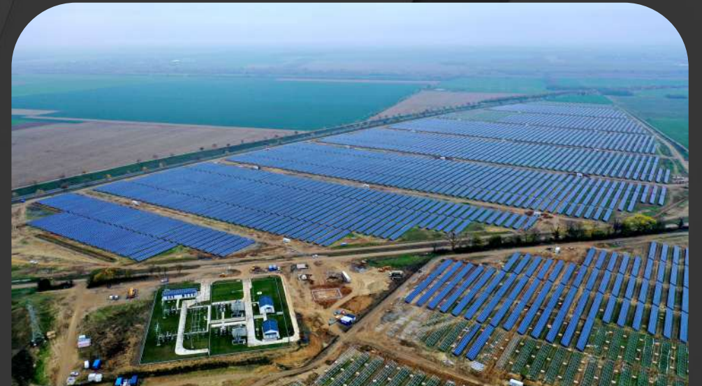
100MW Photovoltaic Power Station Project in Kaposvar, Hungary
