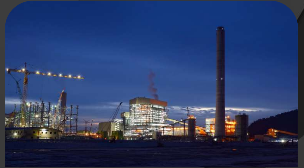
Manjung 1×1000MW Coal-Fired Power Plant Project, Malaysia
