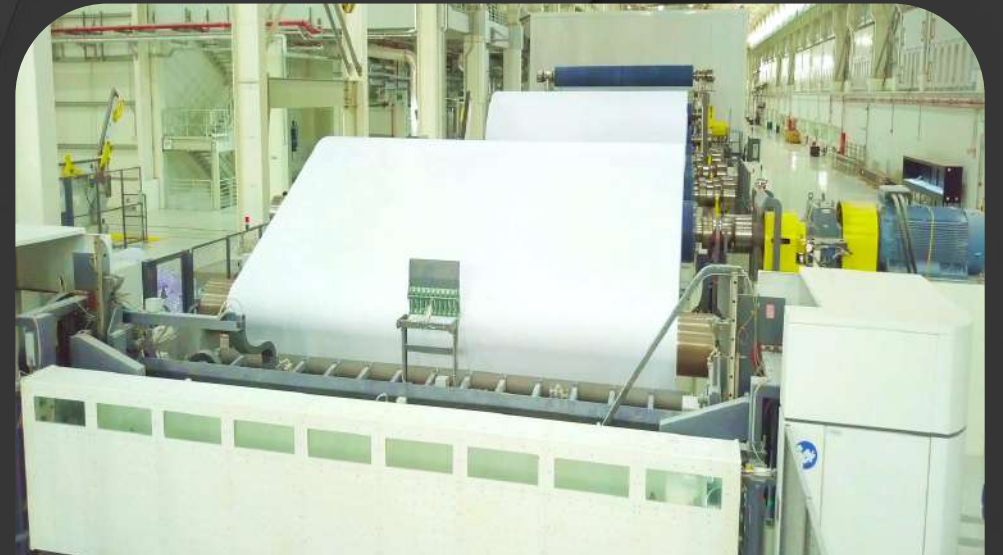
Ittihad Paper Mill Project, UAE
