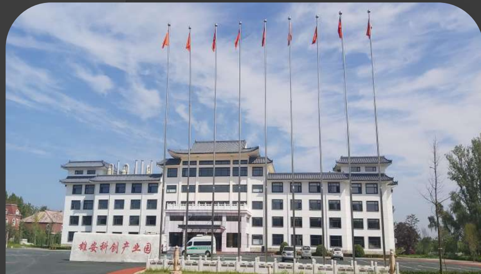
Xiong'an New Area Ecological Environment Bureau Smart Monitoring System (Phase I)
