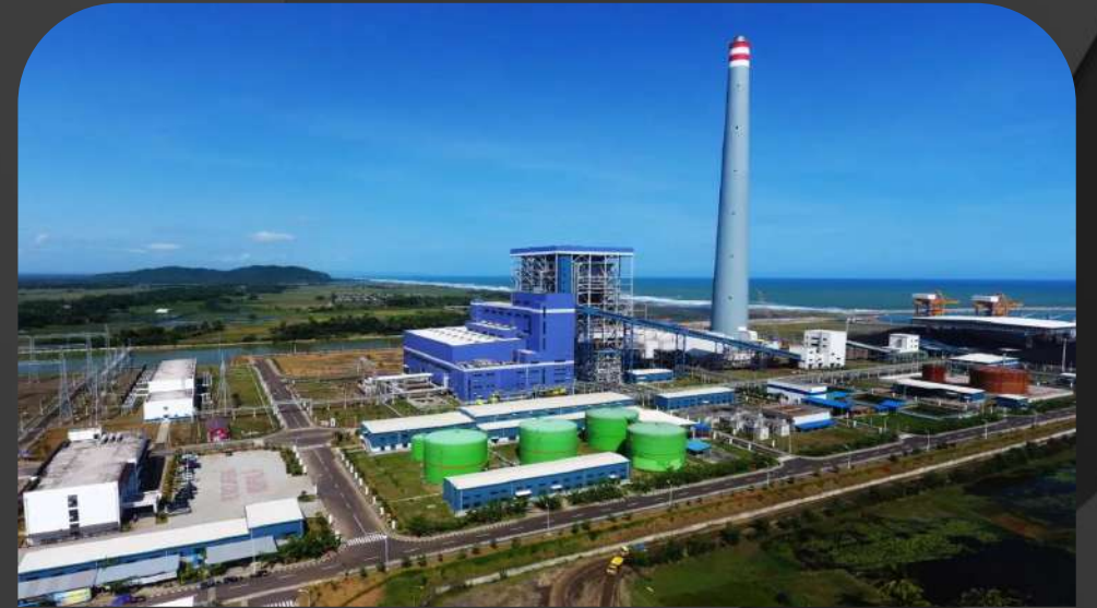
PLTU Adipala Cilacap 1x660MW Super Critical Coal Fired Power Plant Project, Indonesia
